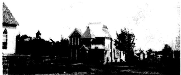
Church - Rail Fence - Dirt Street Corner of Oak and Jefferson
