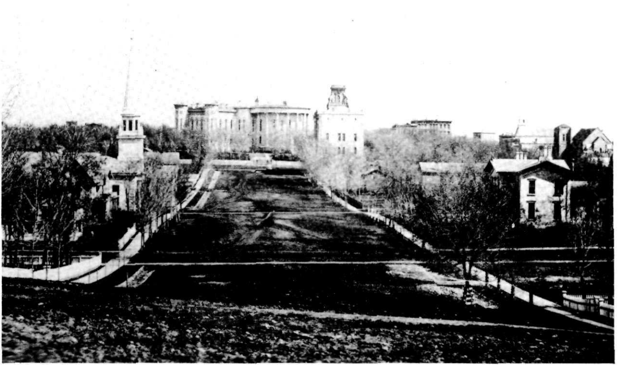
Looking South on Wisconsin Avenue About 1865
