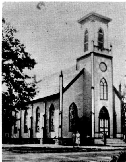
Church with stucco finish after storm had taken off the spire
