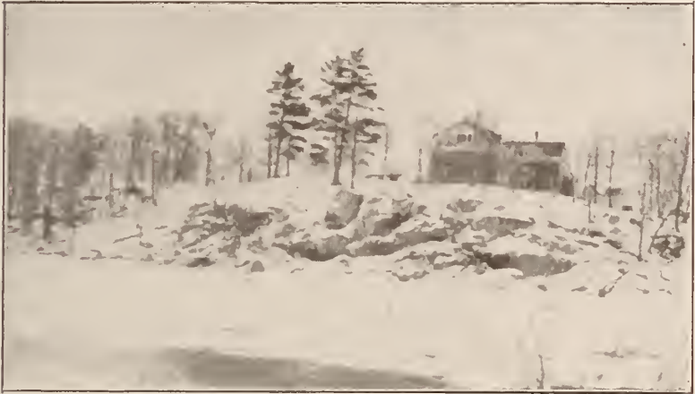
Neillsville Buildings, from West Bank of Black River
